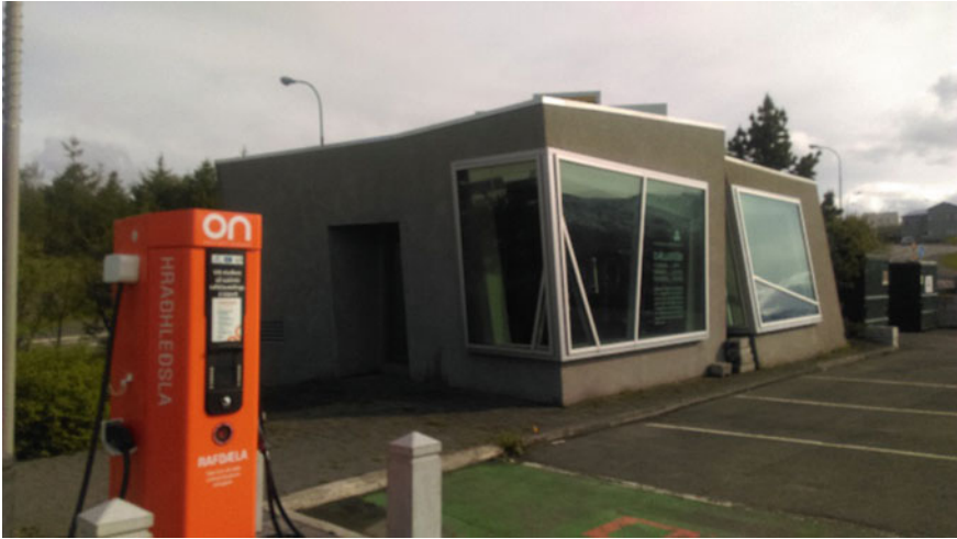
Fig. 21.6 Methane/biogas refilling station
