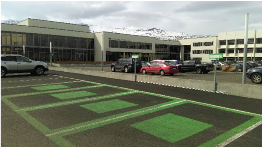
Fig. 21.1 Recharging spots at Akureyri University
